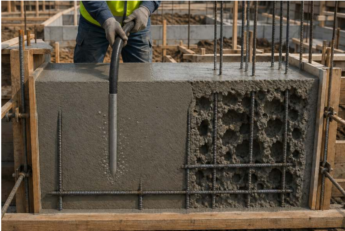
Figure 30. A vibrator helps fresh concrete fill the formwork and release large trapped air pockets
